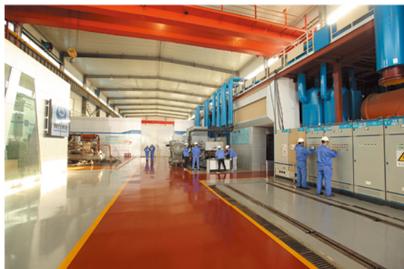
Comprehensive Performance Test Center
