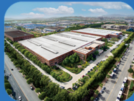
Laishan Industrial Park
